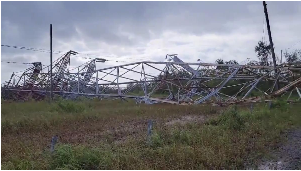
Major transmission tower collapsed near New Orleans
